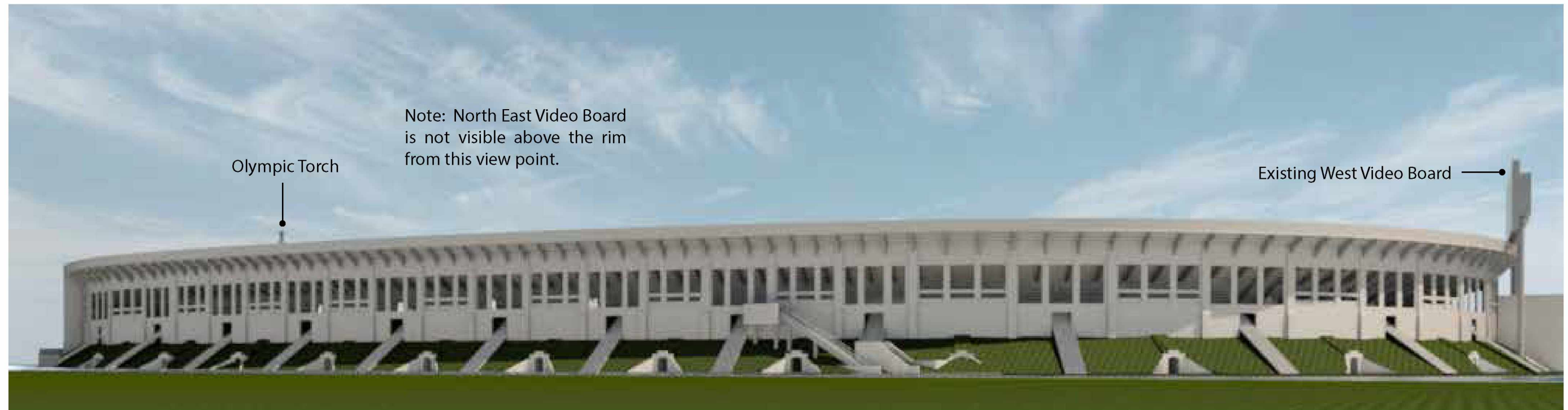
View #1 View from the north side of the Coliseum
