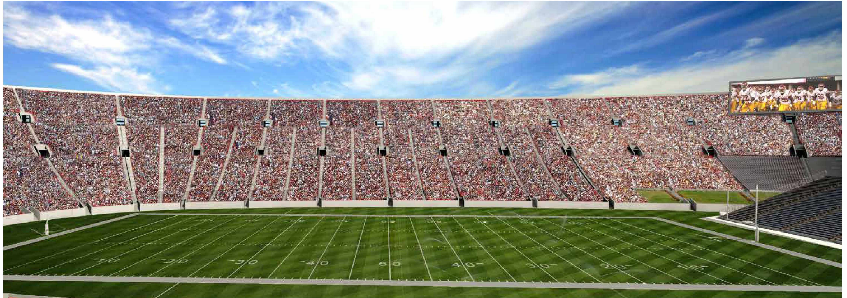
Proposed Bowl Showing Added Aisles and 33" Seating Tread
